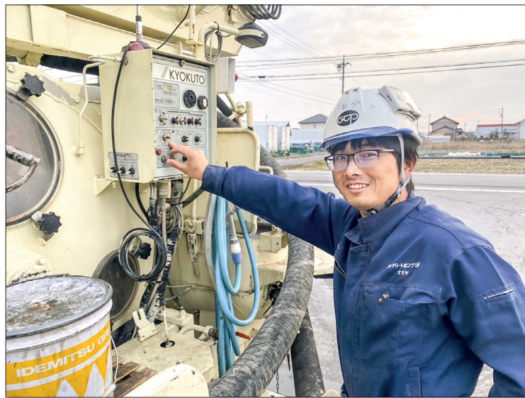
Supplied photo shows Weng Fei, a Chinese national who obtained the Specified Skilled Worker No. 2 status while working at a construction company in Gifu Prefecture, central Japan PHOTO: THE CONSTRUCTION COMPANY/KYODO
