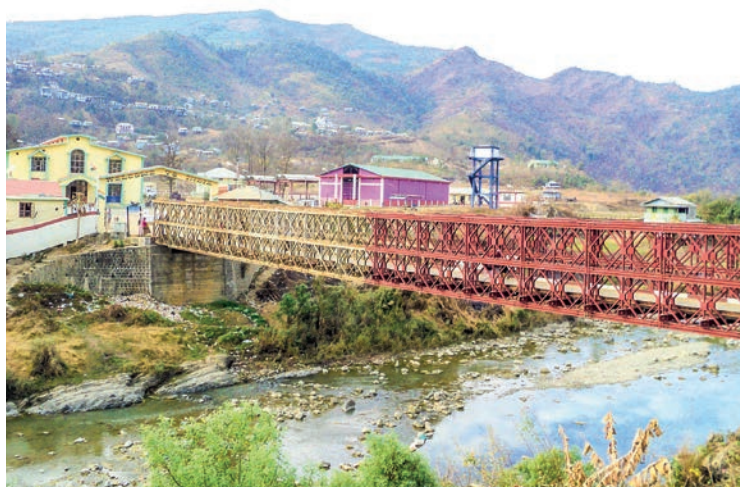
The Reedhorda border bridge between Myanmar and India.
