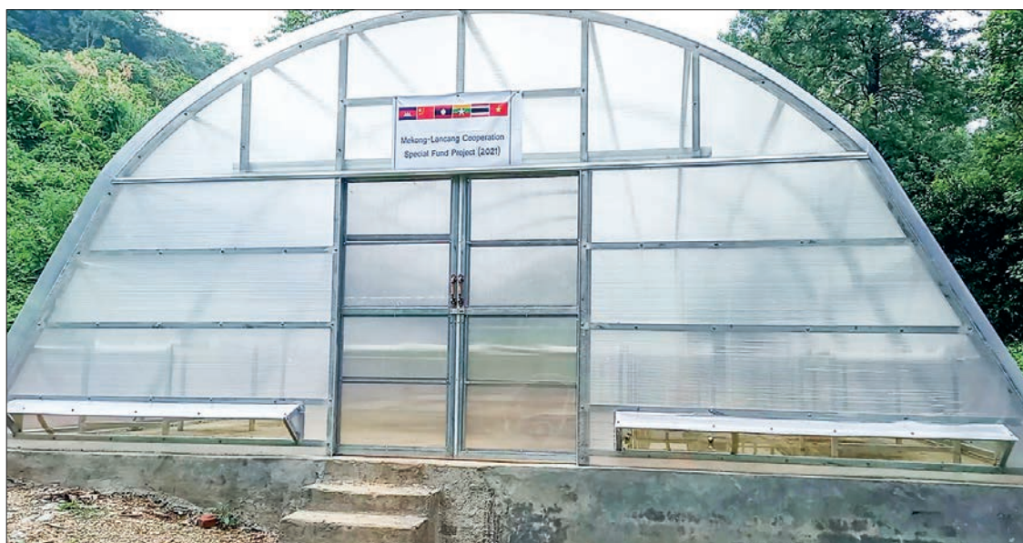
The completed solar dryer.
