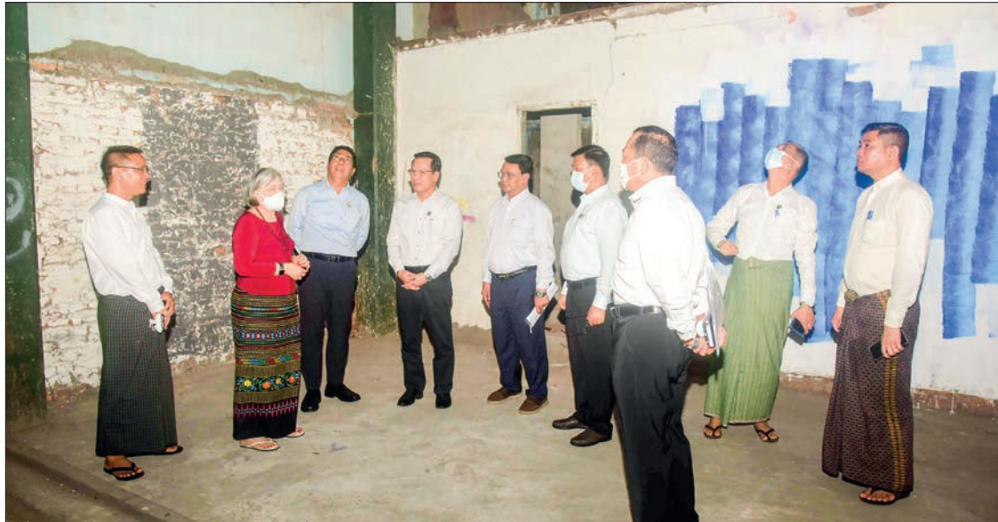
Union Information Minister U Maung Maung Ohn views the upgrading work in the Wazira Cinema.
