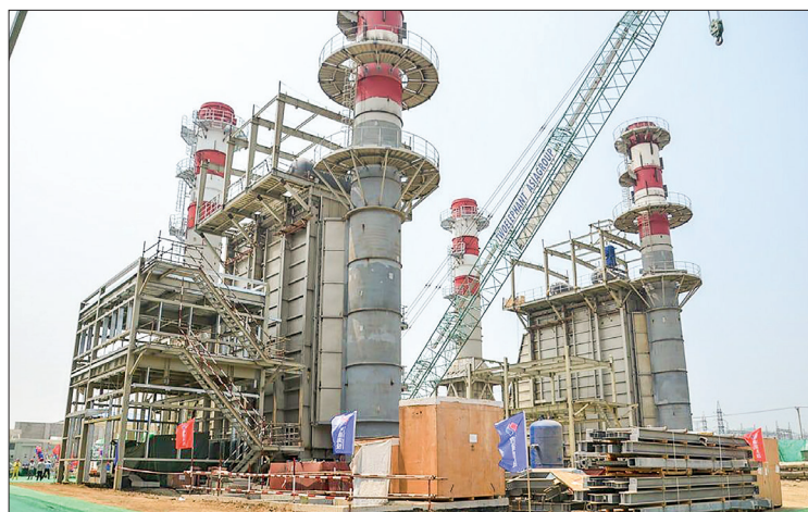
The Kyaukpyu Combined Cycle Power Plant is under construction.
