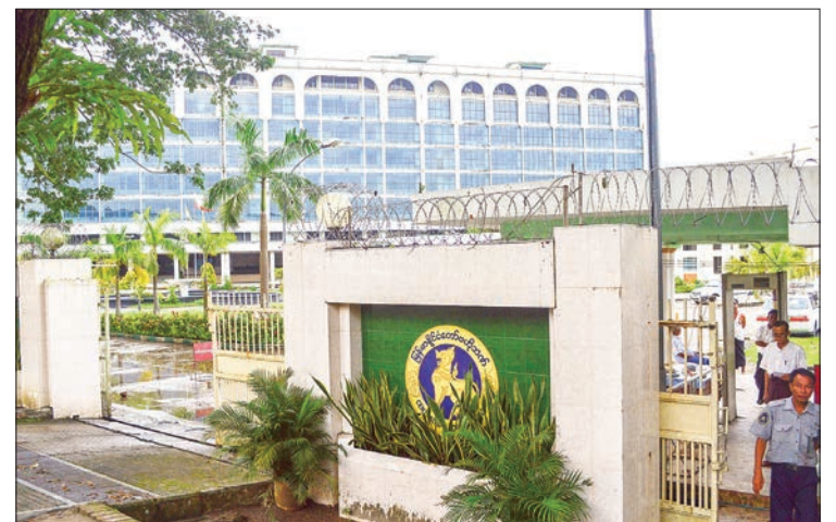
The Central Bank of Myanmar (CBM) building in Yangon.
