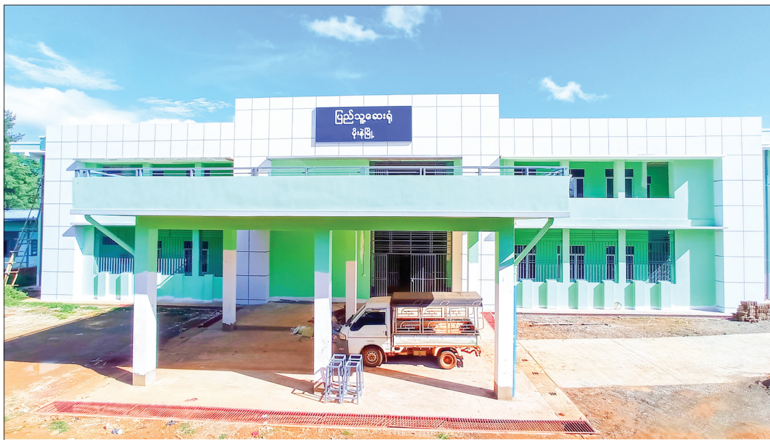
The extended building is a two-storeyed RC building and it is 143 feet in length and 98 feet in width.
