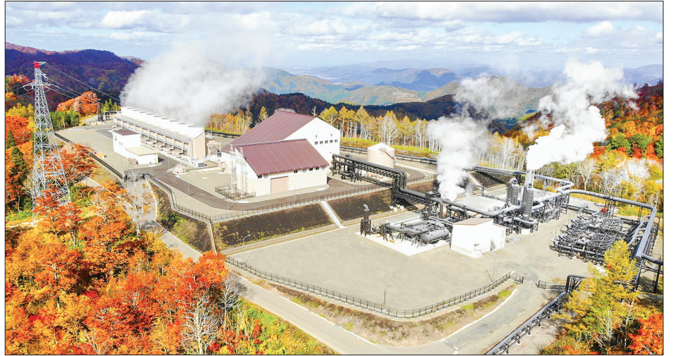
Photo taken in October 2019 shows the Wasabizawa geothermal power plant in Yuzawa, Akita Prefecture. PHOTO: YUZAWA GEOTHERMAL POWER GENERATION CORP./ KYODO
