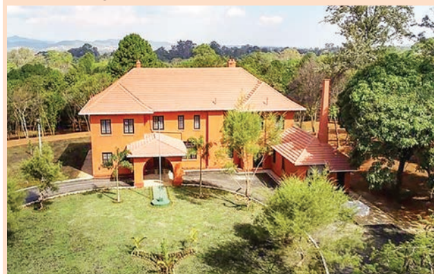
Cherry Myaing: after renovation.
