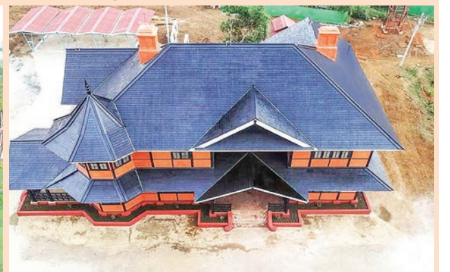
Yuzana Myaing: after renovation.
