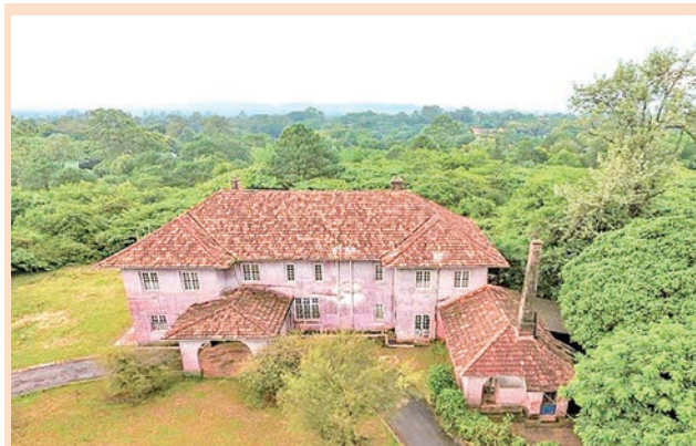
Cherry Myaing: before renovation.
