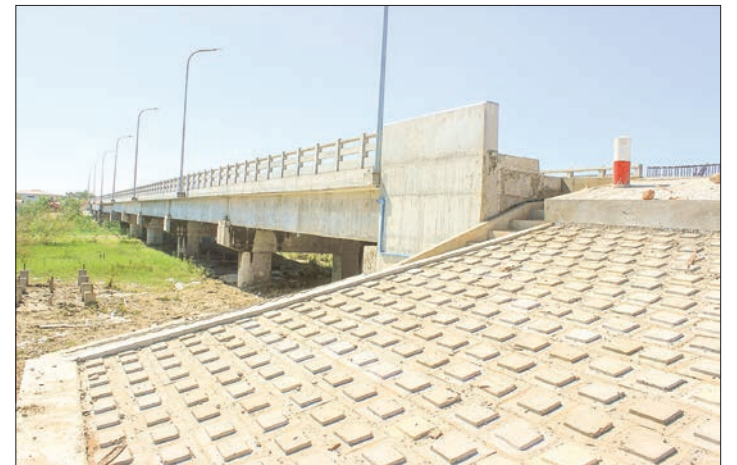
So far, the new Thakhut River Bridge has now completed 100 per cent. The bridge will be able to connect Dala, Kawhmu and Kungyan-gon townships from the Yangon District (South). PHOTO: THUTA
