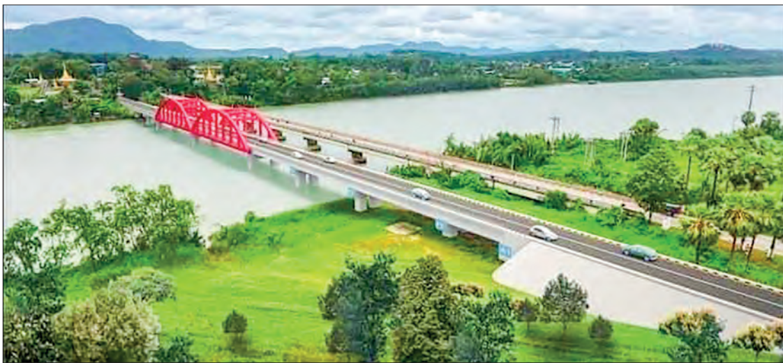
The Kamyawkin Bridge.
