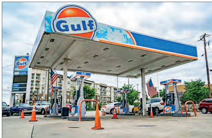
A Gulf service station runs out of gasoline on 11 May 2021 in Atlanta following a hacking attack on the Colonial Pipeline blamed on Russian hackers. PHOTO: AFP/FILE
