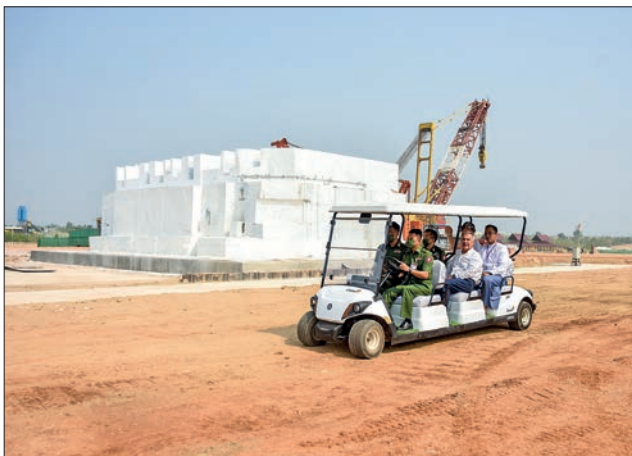
At the construction site of Maravijaya Buddha Image.
