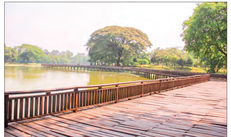
Wooden walkway under maintenance in Kandawgyi Lake.
