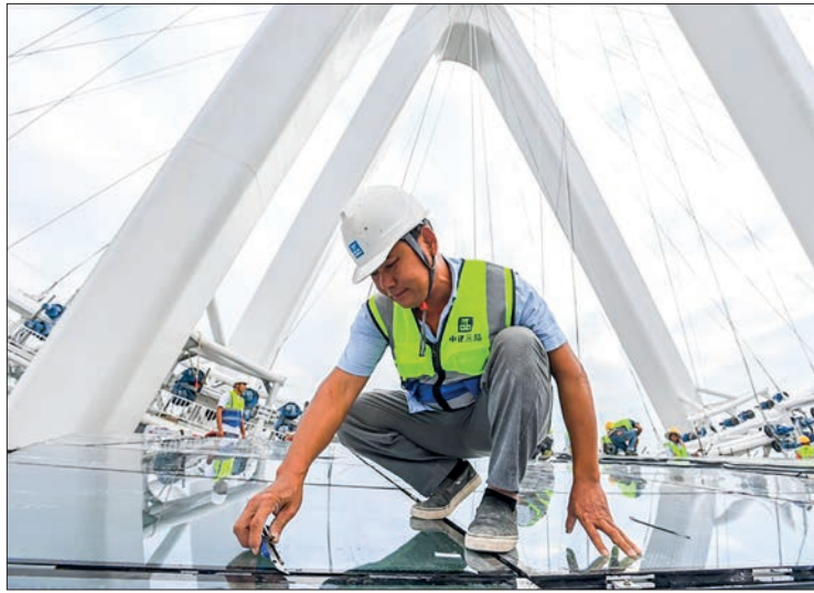
A staff member works at the construction site of a ferris wheel at Baoan coastal cultural park in Shenzhen, south China's Guangdong Province, on 6 Oct 2020. PHOTO: XINHUA/LIU DAWEI
