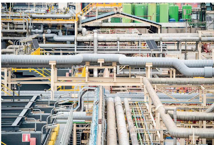
This picture taken on 29 March 2022 shows gas pipelines at the Barcelona's Enagas regasification plant, the oldest in continental Europe, located at the Muelle de la Energia in the port of Barcelona, during a visit for the international press. PHOTO: JOSEF LAGO / AFP
