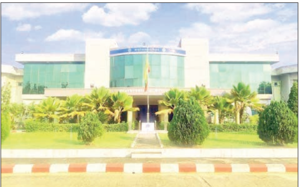
The Ministry of Labour (Head Office).
