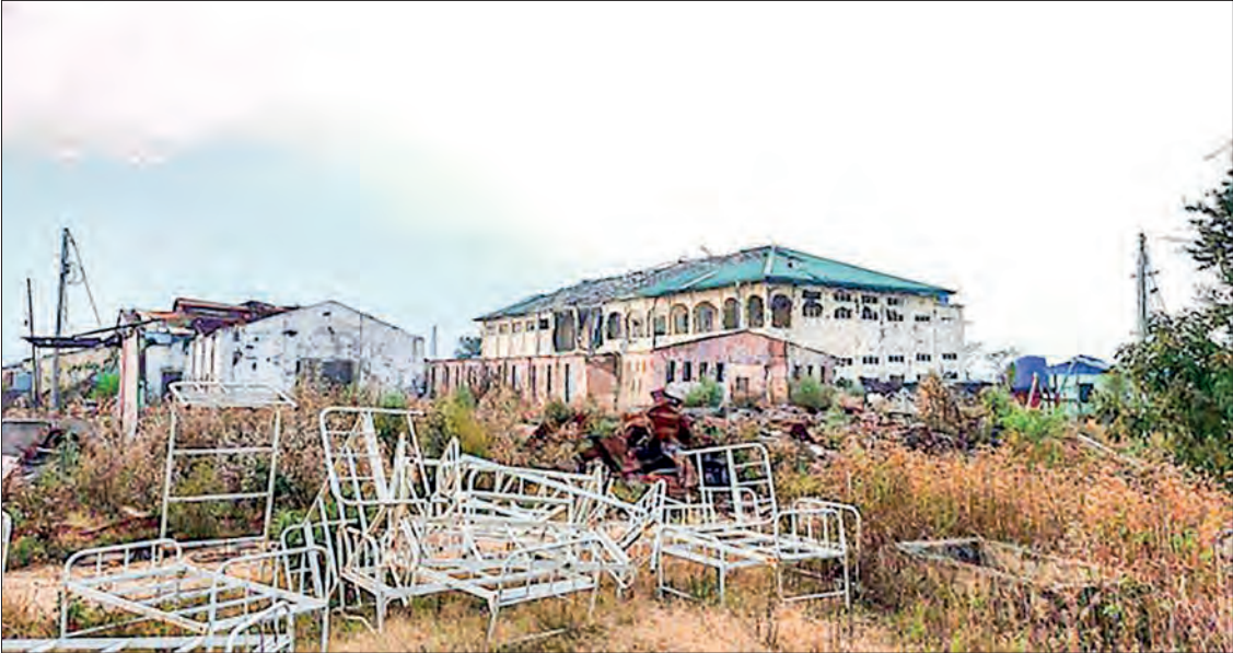
This photo shows the Falam Township People's Hospital which was destroyed by terrorists.
