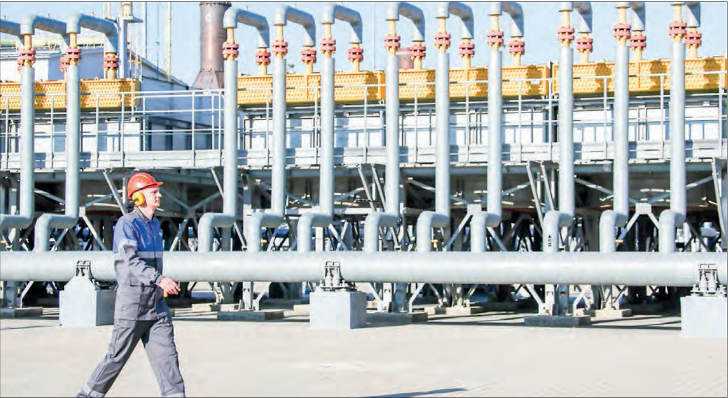
A worker walks by an air gas cooling unit at the Russkaya Compressor Station of the TurkStream gas pipeline in southern Russia’s Krasnodar region. PHOTO: DMITRY FEOKTISTOV / TASS / FILE
