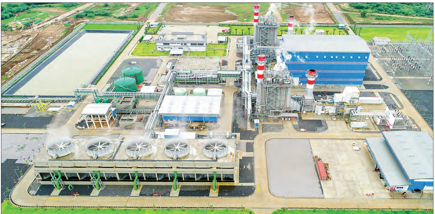
A power plant generating electricity in Myanmar.
