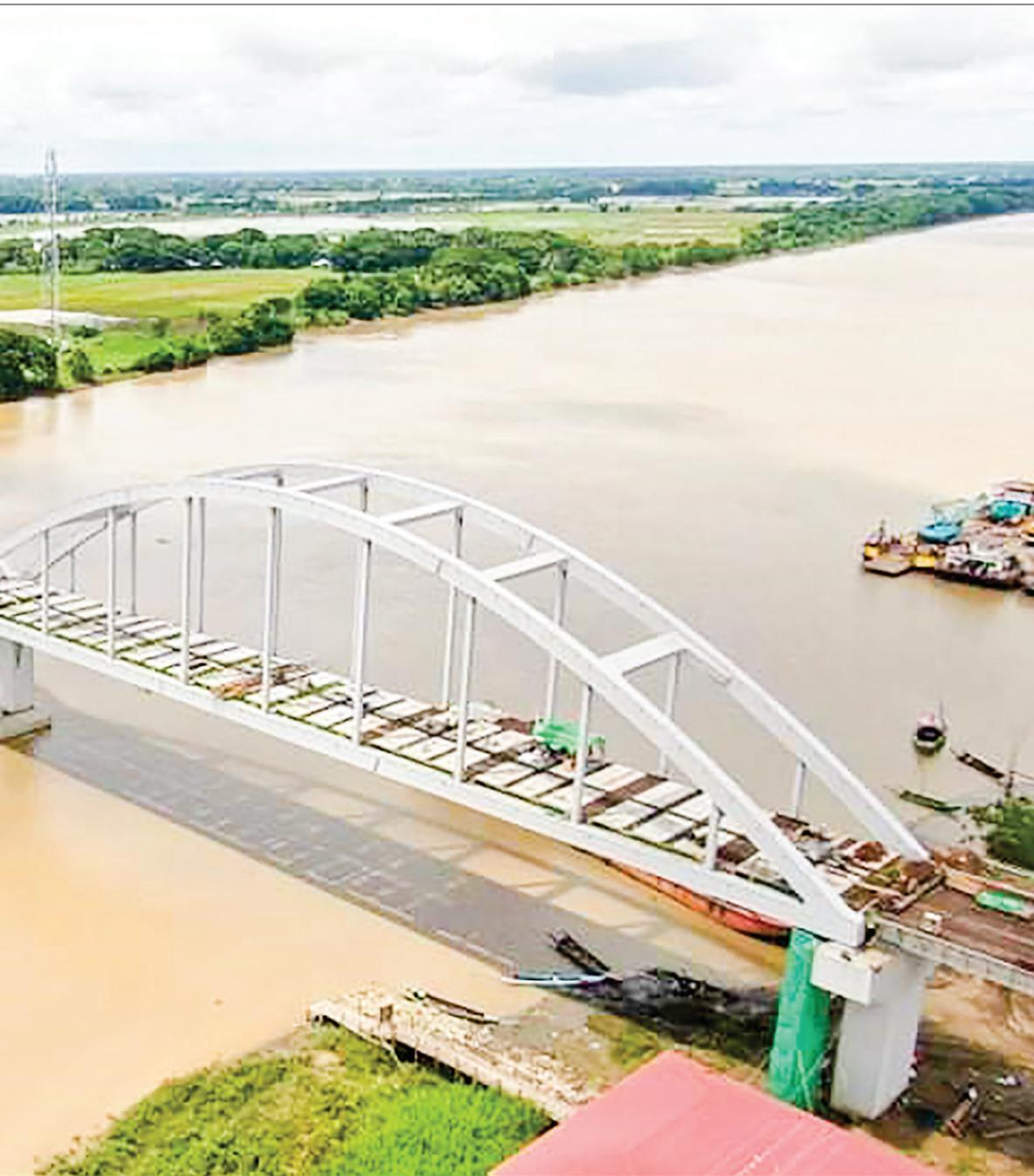
with the floor of reinforced concrete and can withstand up to 60 tons of weight. The bridge's piles are mainly constructed from reinforcement cement concrete and its clearance is 40 ft. and waterway under the facility is 240 ft.
